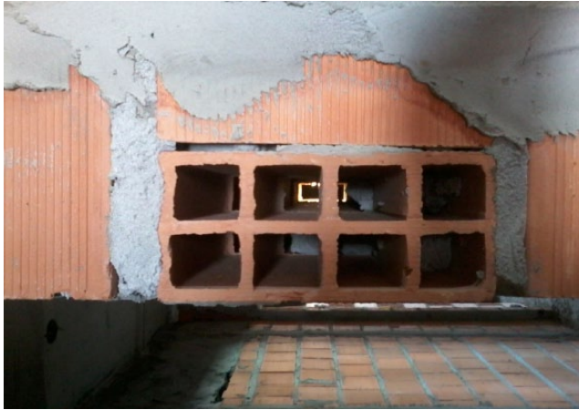
Figure 5. Example of air channels of a ceramic sealing brick.
